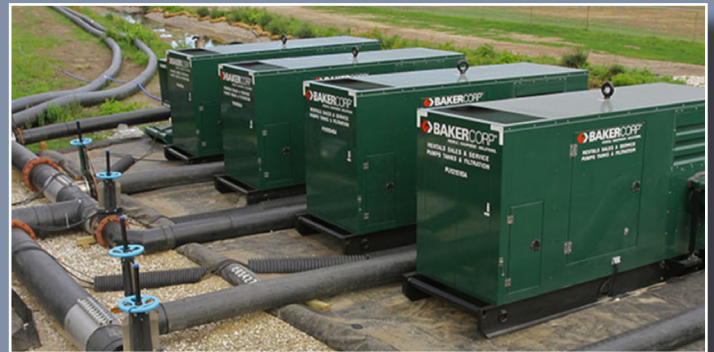
Example of Interim Pumping Facilities, photo courtesy of Baker Corporation
